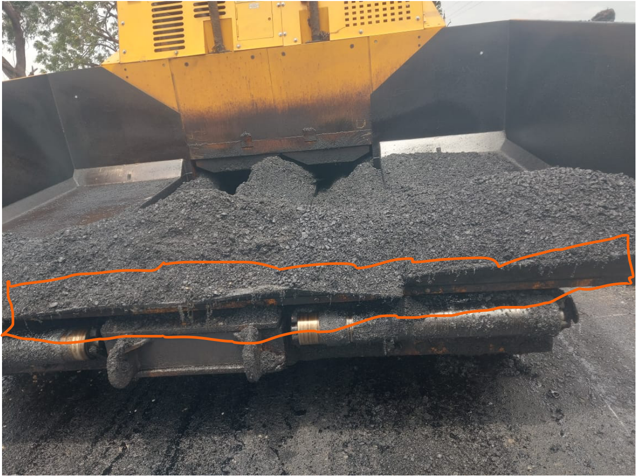
HIGHLIGHTED AREA SHOWS FIBERS IN THE ASPHALT
